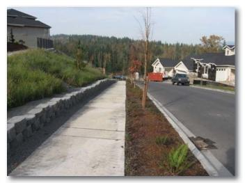
sewer facilities. Site grading was challenged by the natural topography of the site which had areas of relief of more than 150 feet. Accommodation of the existing grade in the developed condition required significant structural walls with consideration of access to golf course amenities, existing trail systems, and view potentials.
